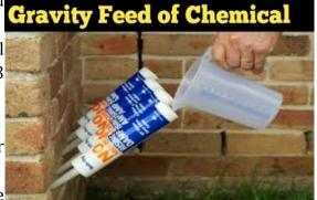
Fig 1.11 Gravity feed of chemicals
