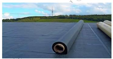
Fig 1.8: EPDM Waterproofing Membrane
