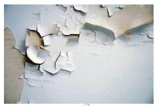
Fig 1.15 Flaking defect
