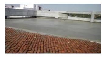
Fig 1.9 Brick Bat Coba Waterproofing
