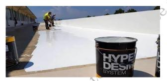
Fig 1.5: Polyurethane liquid Membrane
