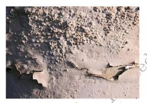
Fig 1.12 Peeling Defect
