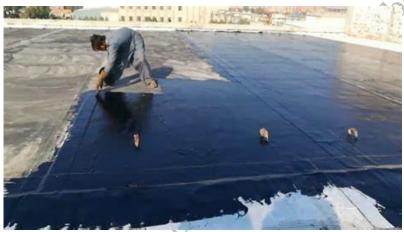
Fig 1.4: Bituminous Coating Waterproofing
