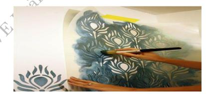
Fig 3.1 Painting using stencil
